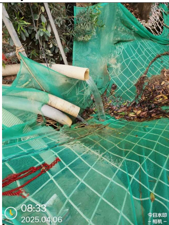
Photo 3-10 Discharge point of Silt Removal Facility at Portion E3
