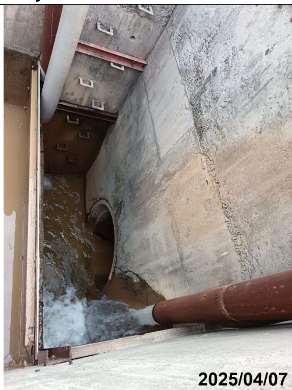
Photo 3-12 Discharge point of Silt Removal Facility at Portion B2/E1
