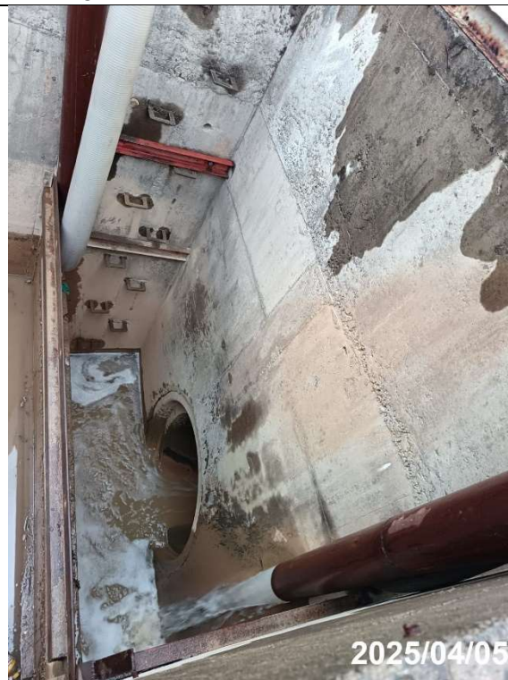
Photo 3-5 Discharge point of Silt Removal Facility at Portion B2/E1
