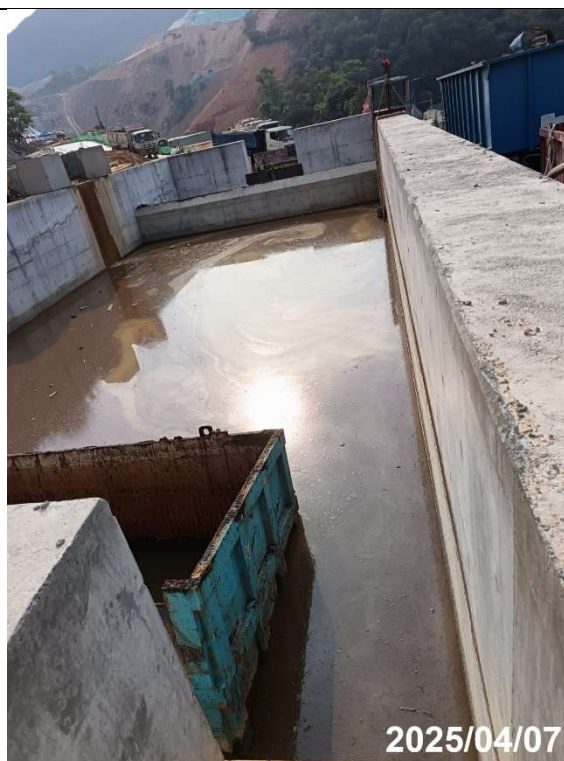
Photo 3-11 Sedimentation Basin at Portion B2/E1
