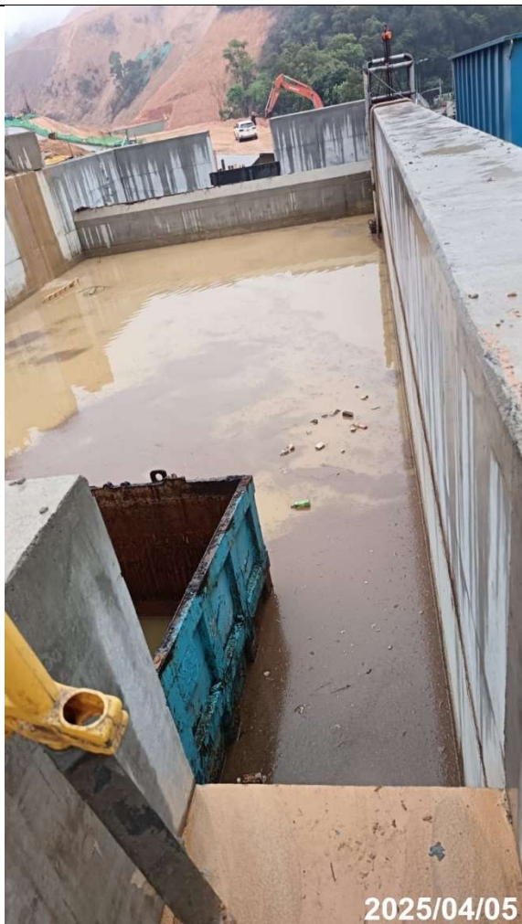
Photo 3-4 Sedimentation Basin at Portion B2/E1
