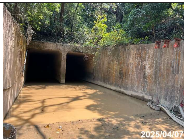
Photo 3-16 River confluence position between the Box Culvert under Wo Keng Shan Road and Branch of Existing Channel near Portion A
