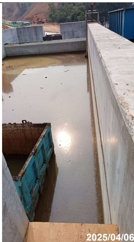
Photo 3-7 Sedimentation Basin at Portion B2/E1
