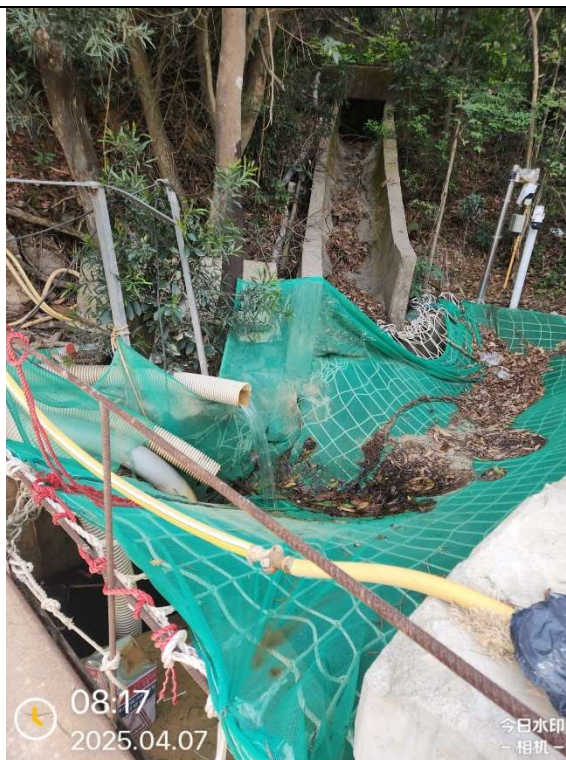
Photo 3-14 Discharge point of Silt Removal Facility at Portion E3
